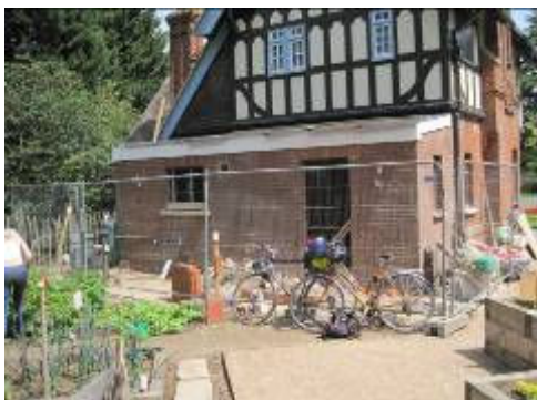
Working around the lodge refurbishment
